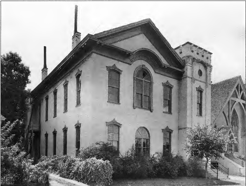
SEVENTEENTH WARD CHAPEL BUILT IN 1874, 149 WEST 200 NORTH (THEN 100 NORTH) STREET. RENTED FOR LDS COLLEGE USE 1895 – 1897.
